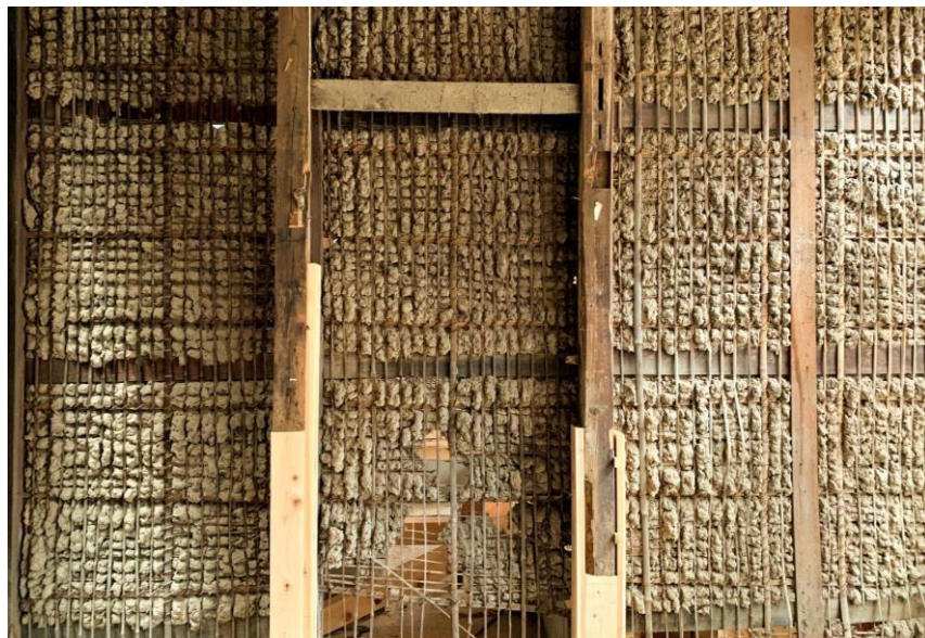
補強後の柱と土壁の下地 Reinforced Columns and Framework of Earthen Wall
